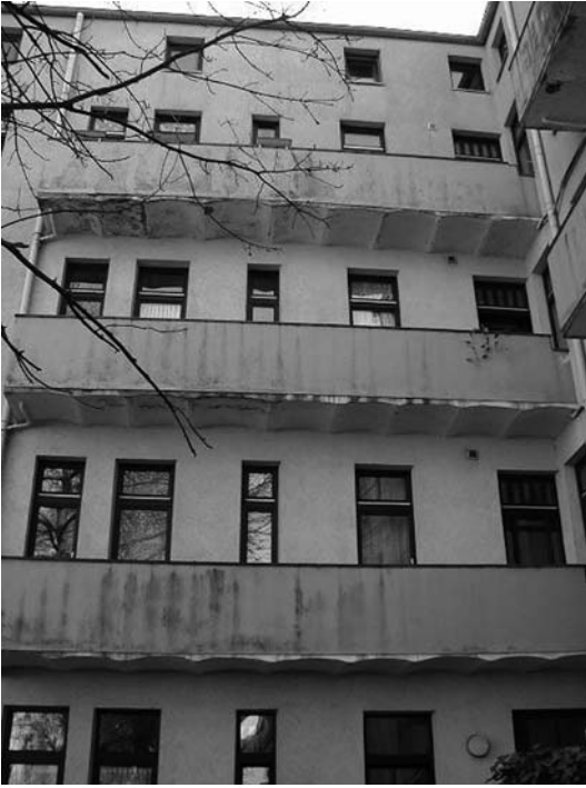
Figure 9. The dilapidated building underwent a complete renovation, including an elevator addition to create an accessible building. The old balconies ( left ) were removed and new balconies added for private outdoor space. ( Source : Ståwog)
