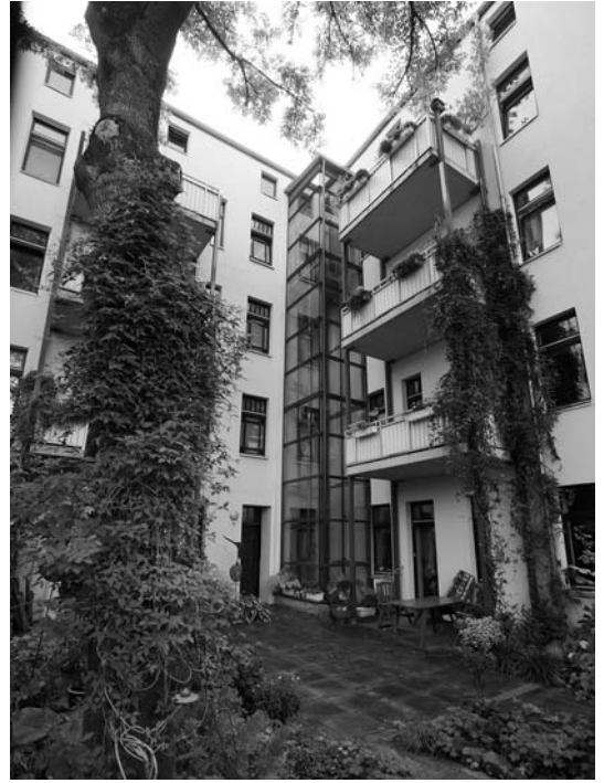
Figure 9. The dilapidated building underwent a complete renovation, including an elevator addition to create an accessible building. The old balconies ( left ) were removed and new balconies added for private outdoor space. ( Source : Ståwog)
