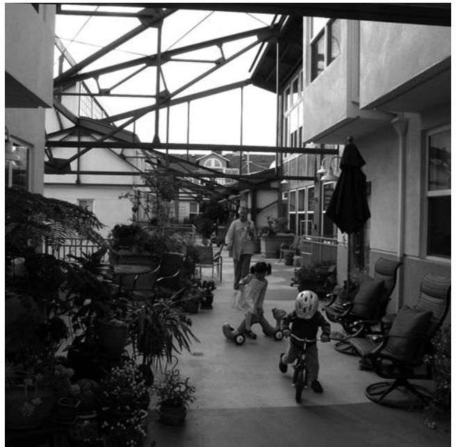
Figure 5. The narrow central pedestrian street separating the two rows of units works well and allowed the housing to fit within the framework of the historic trusses.
