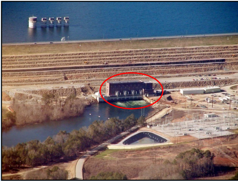
Dam and hydroelectric powerhouse
