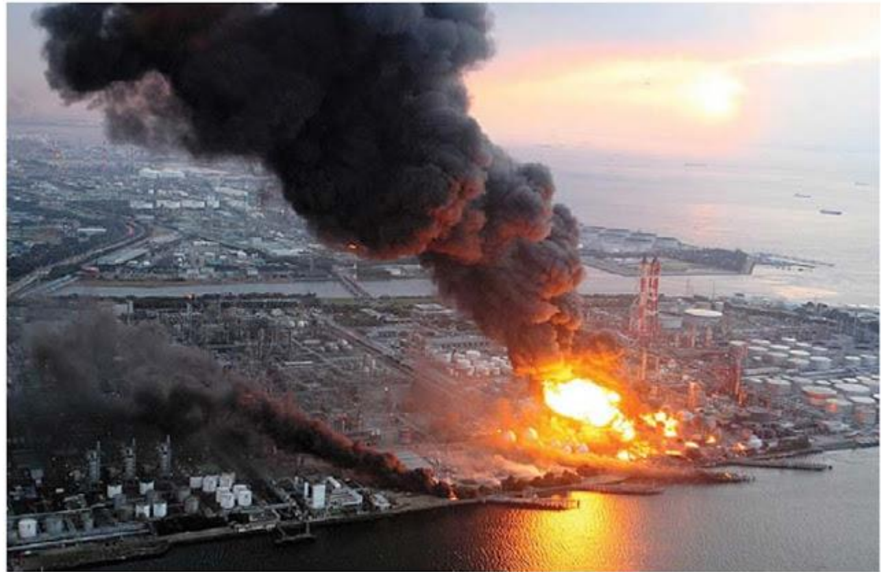
Broken gas tanks erupt in fountains of flame after the 2011 Tohoku, Japan, earthquake.
