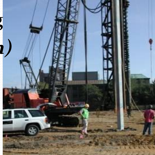
A pile driver sets the stage for construction.
