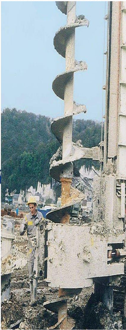
(a) Drill into caving soil and add slurry as necessary for adequate head and to required depth.
